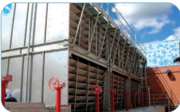
Basinless Series 3000 Cooling Tower on a concrete basin
