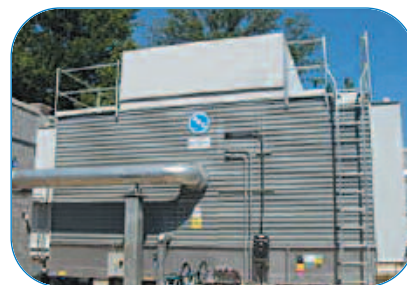
Unit with intake and discharge sound attenuation
