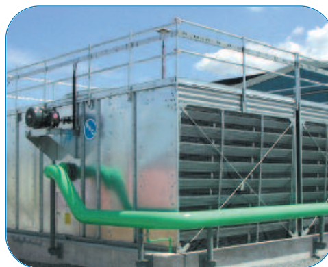
Gear drive system, externally mounted motor
