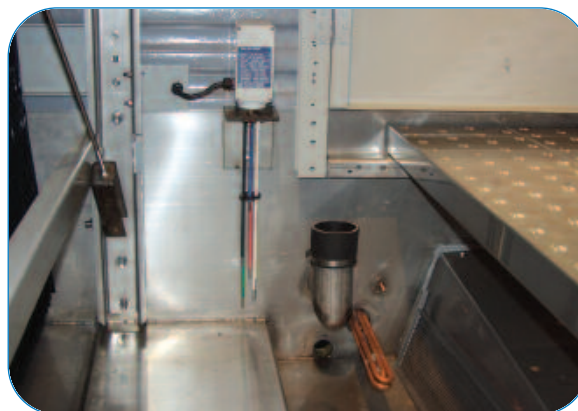
Electric water level control package & basin heater
